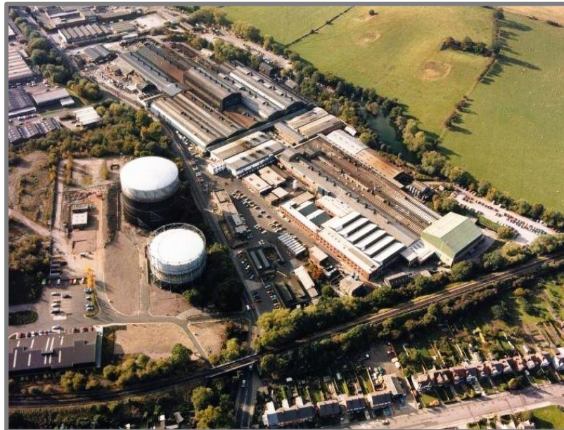
Aerial view showing factory and gasometers
