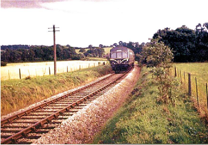
Above – Train near Oakenshaw Farm Below – Lapworth Station
