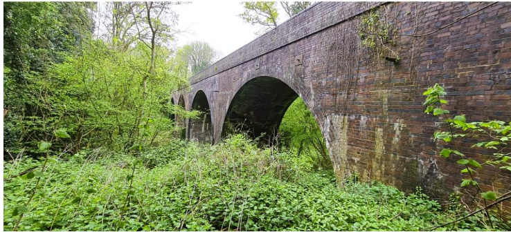
The Broad Dingle viaduct, just north of Alfrick, still stands on the parish boundary with Lulsley as a testament to the hard work of the navvies. Our man may have been involved in the construction in the months before his death.
